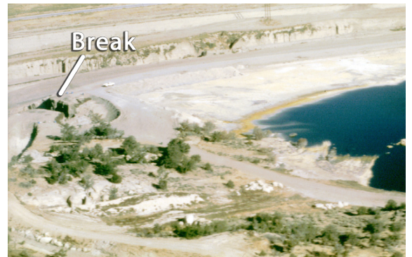
Photo of the break in the dam where the tailings flowed through. The yellow "beach" on the tailings is sulfur, not yellowcake.
